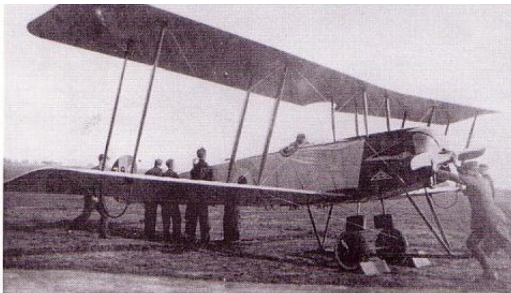
The Avro 504D, only six of which were built, was the RFC version of the 504C but with a comma style rudder. The first 504D was delivered in August 1915.
